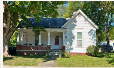
1705 S Campbell Street Hopkinsville, KY
